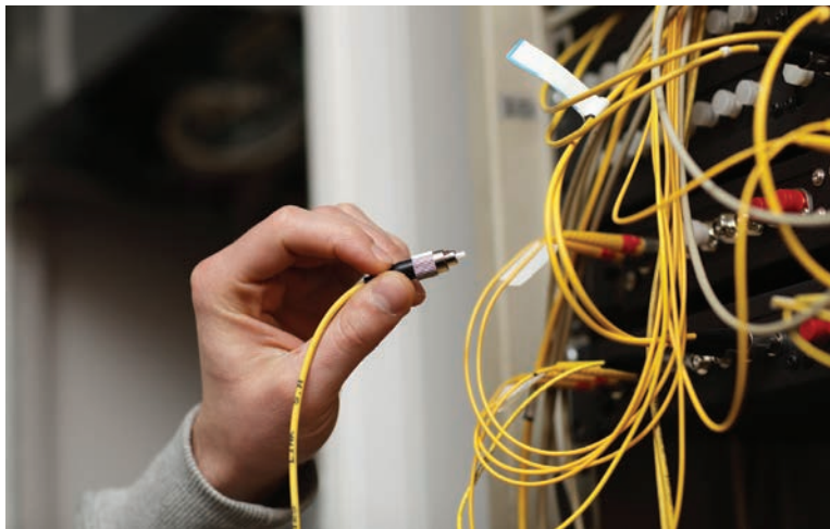
Photo 1. Technician attaching fiber optics
